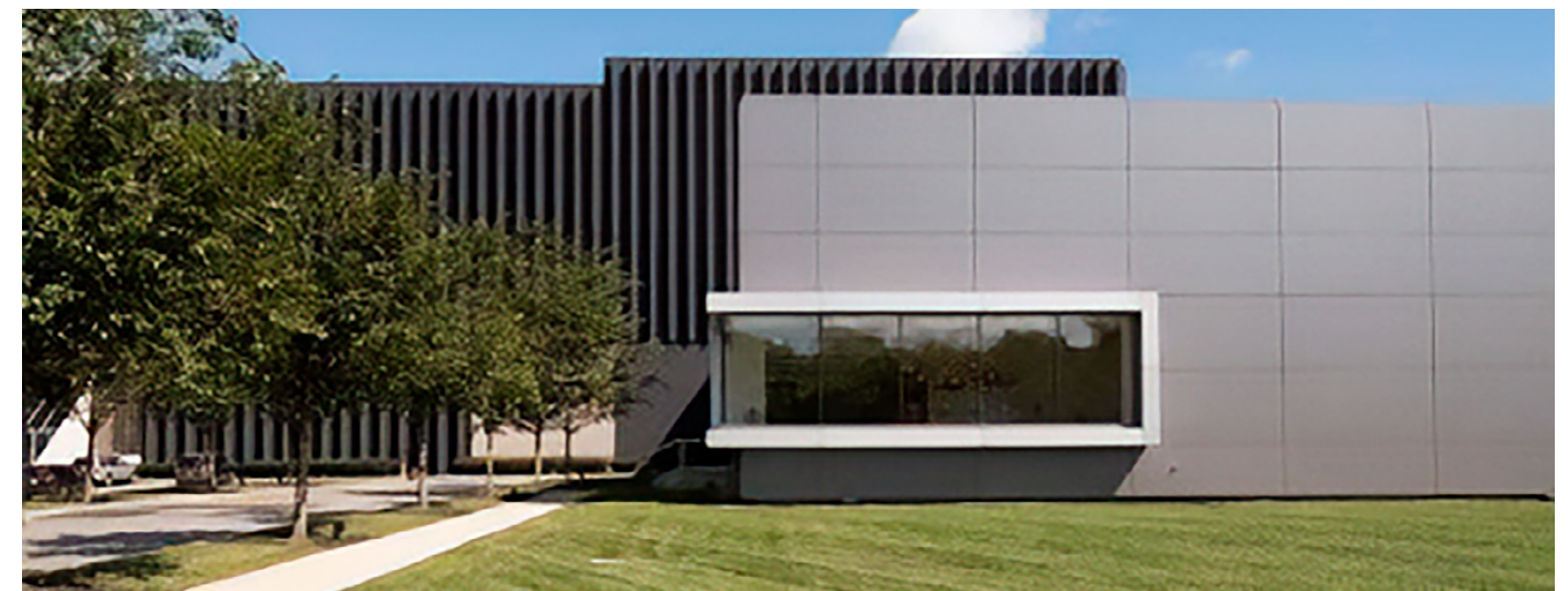
Markley data center in Massachusetts
